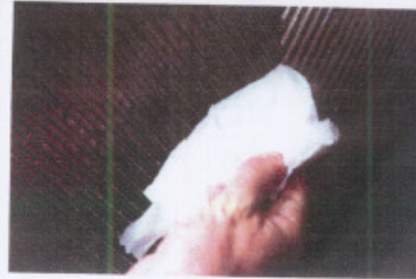
Aifa-laval exchanger Quench water side Mat polymeric sediments may be removed from plate surface by soft paper.
